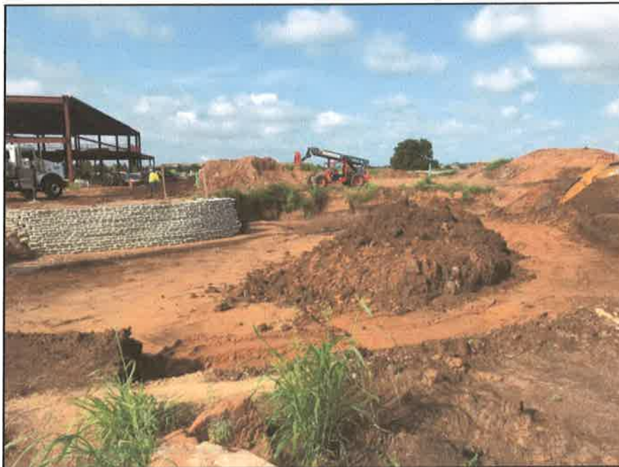
Photo 8: Wall Stabilization and Over-dig in Southwest Excavation Block, Facing Southwest.
