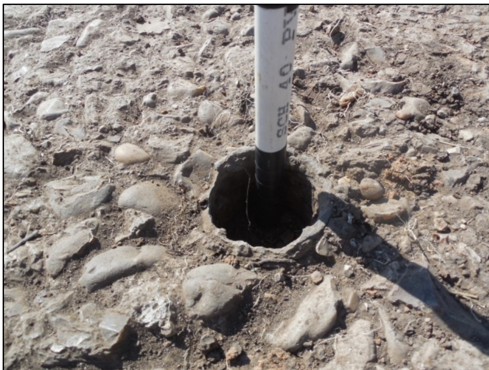
Figure 4.10: Feature 13, Well with Concrete Base and 7.6-Centimeter-Diameter Standpipe, Metric Scale in 10-Centimeter Increments
